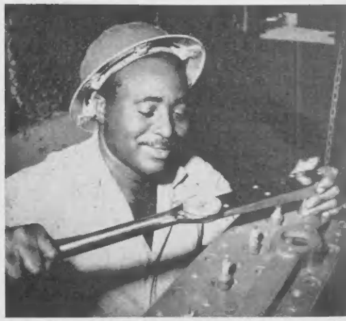
BOLTS ARE tightened through the use of a foot-pounds torque wrench. BOLTS TA worde cerrá usando un yabi di torque cu ta marca foot pounds.
